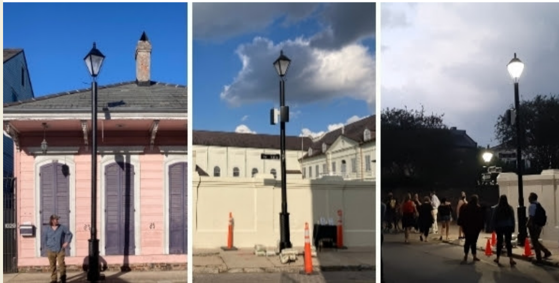
Toro Blanco's 20 foot 5G pole modeled after existing French Quarter streetlights.
